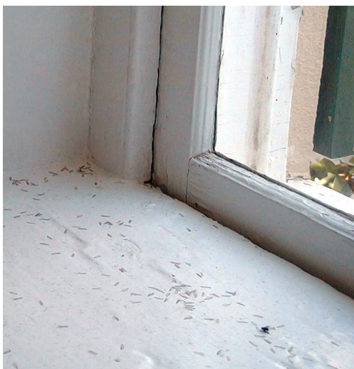
Figure 8. Shed wings on a window sill are a sign of infestation. (B.T. Forschler)
